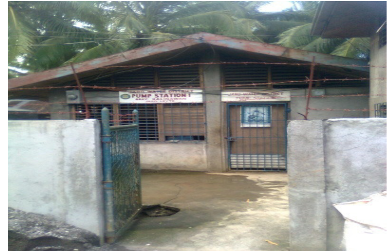
✓ PUMPING STATION #1 (DEEP WELL): CAPACITY 10 LPS SUBMERSIBLE PUMP
